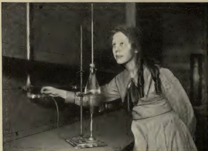
FIG. 42. A thermometer made of a flask of water. It does not show the exact degree of heat of the water, but it does show whether the water is hot or cold.
